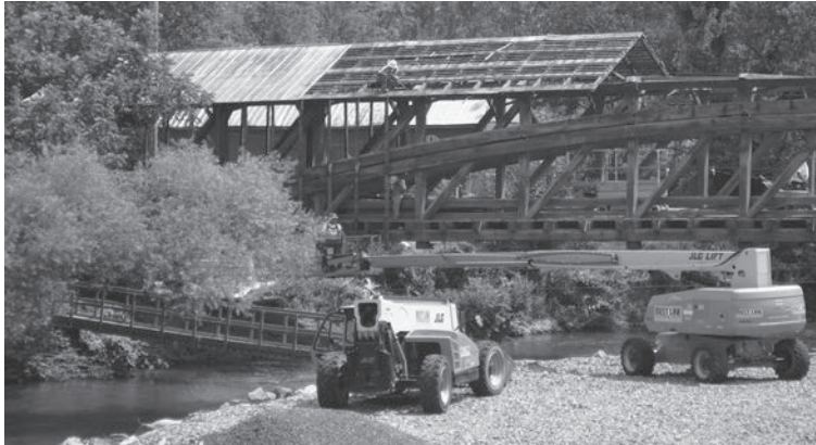
Siding is all gone and roof removal in progress.
