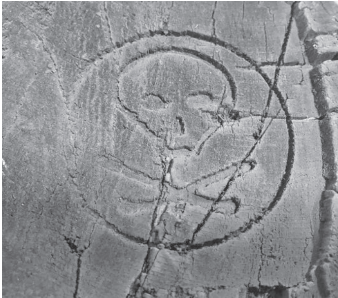
"Poison" warning stamped on beam from Dreibelbis bridge. Poison was used to keep bugs and critters from chewing on it.
