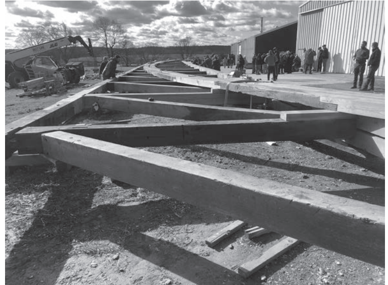
One side wall with Burr Arch. Beams that are lighter color are ones that have been replaced.
