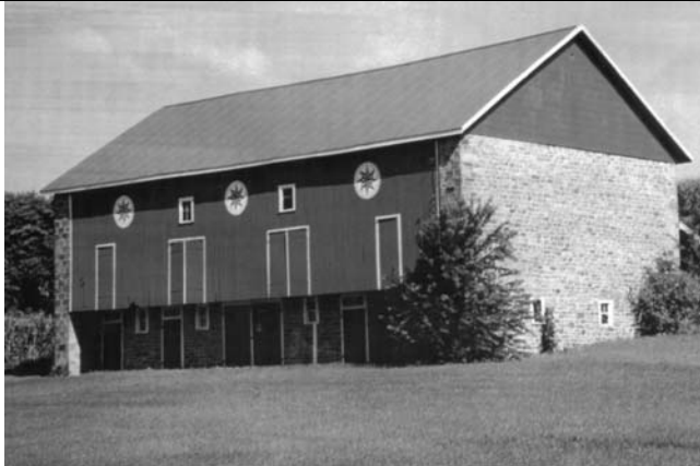
Dreibelbis Homestead - barn has recently been repaired by Giorgi Mushroom, current property owner. As funds permit, they plan to restore the remainder of the buildings. Giorgi also maintains the lawn areas. Across the road is where the Dreibelbis Spring was located and from which Abraham's Mill got its power. The volume was such that there were trout in the stream.
